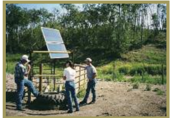
Solar powered remote watering system for livestock, August 2002
